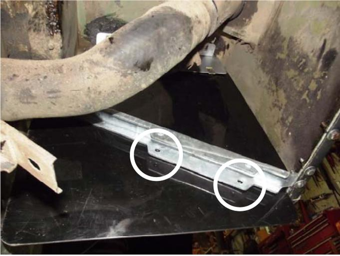
Now fit the mud shield in place. Mark out the two holes to be drilled, make sure the mud shield doesn't rub the side panel, leave a slight gap. Remove the shield and drill the two holes (circled) with an 8mm drill bit.
